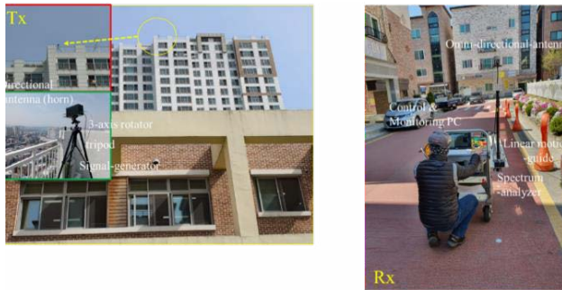
Fig. 4. Fabrication of the installed Tx (left) and Rx (Right)
